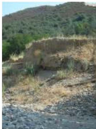
2—Unnaturally high eroded berm, possibly from track construction.
