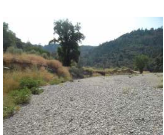
3—Eroded river bank, over 100’ long with drainage pipes protruding.
